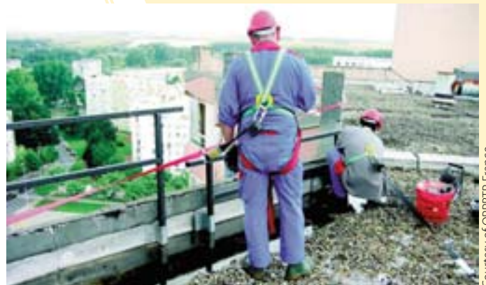
Courtesy of OPPBTP, France
